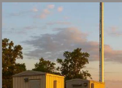
Telecom Shelters & BTS Sites
