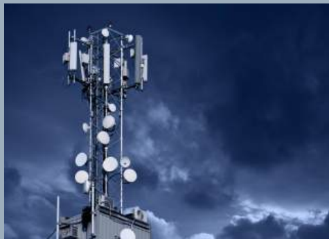
5G & LTE Towers
